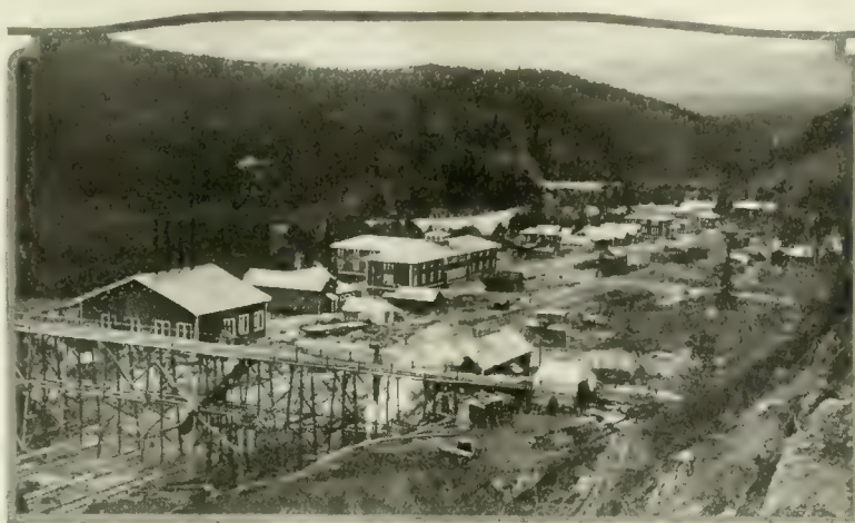
View of the Chickaloon coal field in Alaska, showing mining operations carried on by the Navy Department before supervision of the fields was transferred to the Department of the Interior
